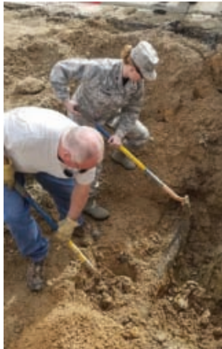
Maj. Perronne and Robert Bringhurst excavate a broken water main.
