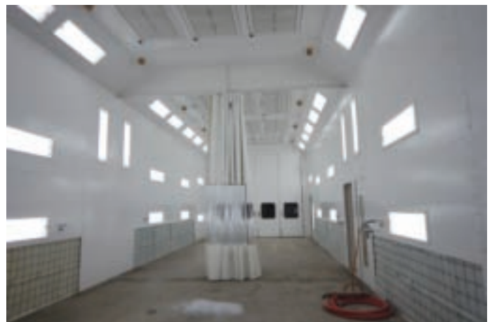
New Consolidated Support Maintenance Shop paint booth at the Draper headquarters.
