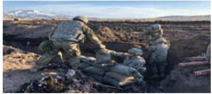
The 116th Engineer Company Soldiers prepare trenches with individual fighting positions to fortify their patrol base.
